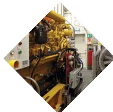
Detail of 3516B genset with local panel & preheating system.
