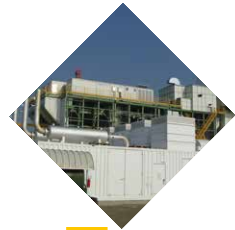
Seven 3512B drilling genset into sound attenuated Containers.
