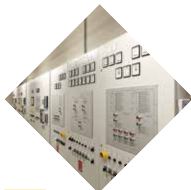
Detail of Control Room with Unit Control Panels & Master paralleling control panels.
