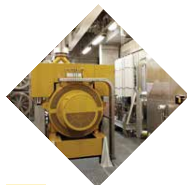
Detail of Power Generation room & MV alternator.
