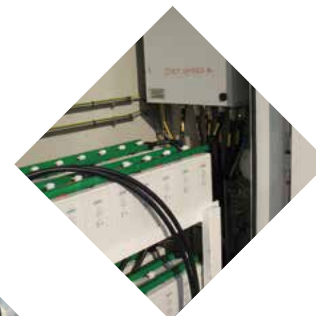
Ni-Cd starting batteries.
