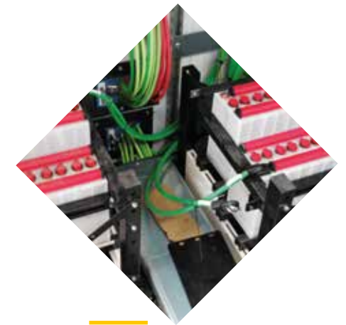
Ni-Cd Starting Batteries.
