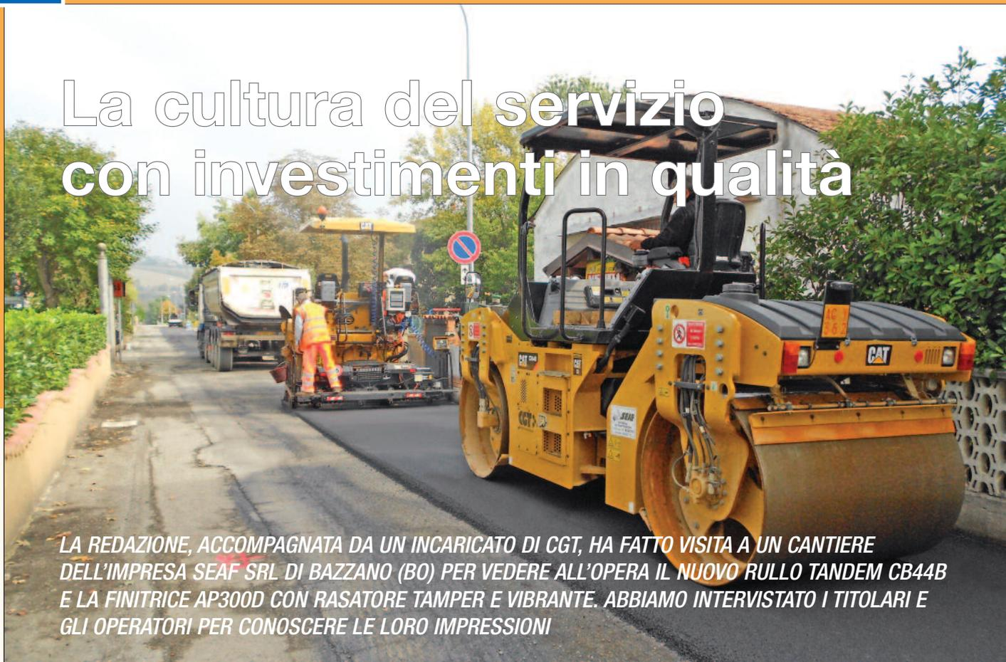
LA REDAZIONE, ACCOMPAGNATA DA UN INCARICATO DI CGT, HA FATTO VISITA A UN CANTIERE DELL'IMPRESA SEAF SRL DI BAZZANO (BO) PER VEDERE ALL'OPERA IL NUOVO RULLO TANDEM CB44B E LA FINITRICE AP300D CON RASATORE TAMPER E VIBRANTE. ABBIAMO INTERVISTATO I TITOLARI E GLI OPERATORI PER CONOSCERE LE LORO IMPRESSIONI
